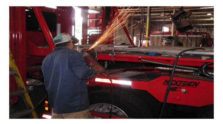
STEP 4: INSTALL NEW GUSSET ¼" OFF THE EDGE OF THE CATWALK. WELD 50%.
